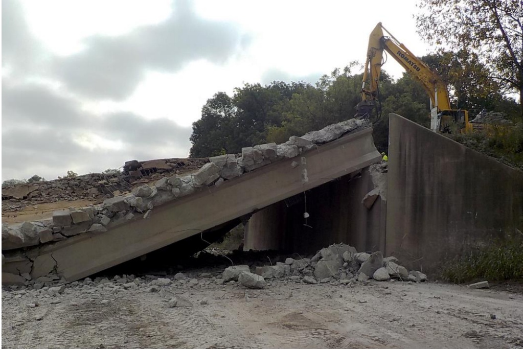
Photo of mechanical demolition/removal of an existing interchange concrete beam single span bridge that was part of the old/previous SR 422 highway.
