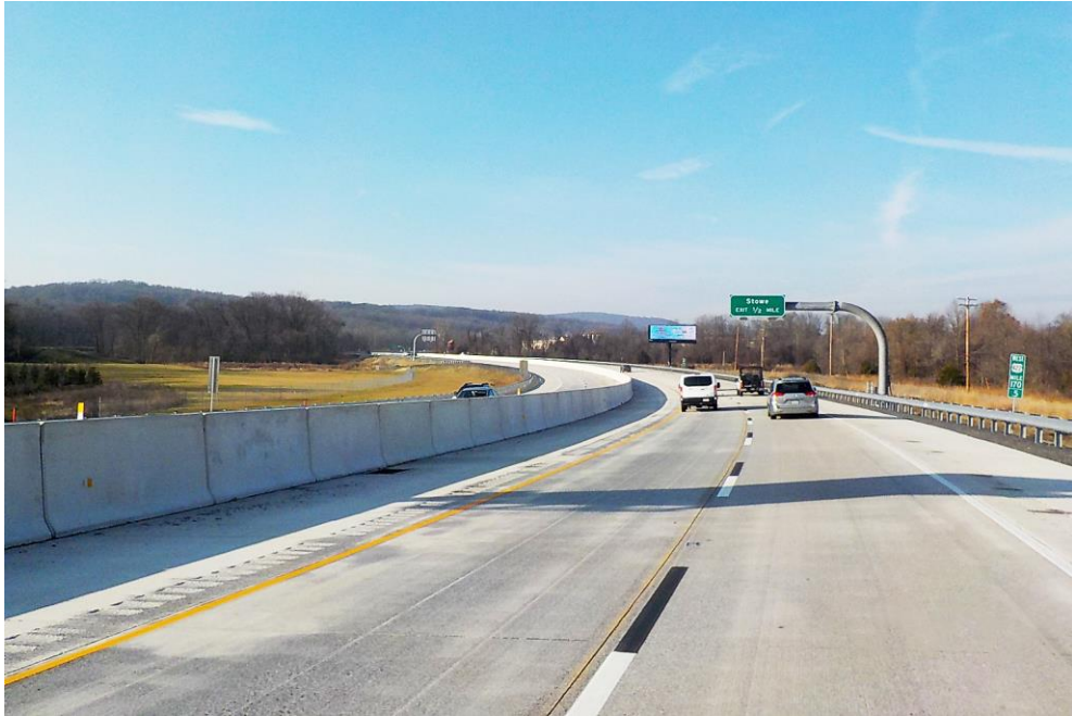
Photo on SR 422 looking westward at start of the highway realignment, where old SR 422 was removed to provide an open flood plain along the Schuylkill River.
